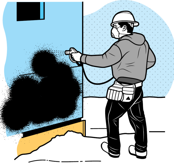
LIQUID VAPOR BARRIERS ARE SPRAYED ONTO THE EXTERIOR OF A HOME TO MAKE IT AIR AND WATER TIGHT.
