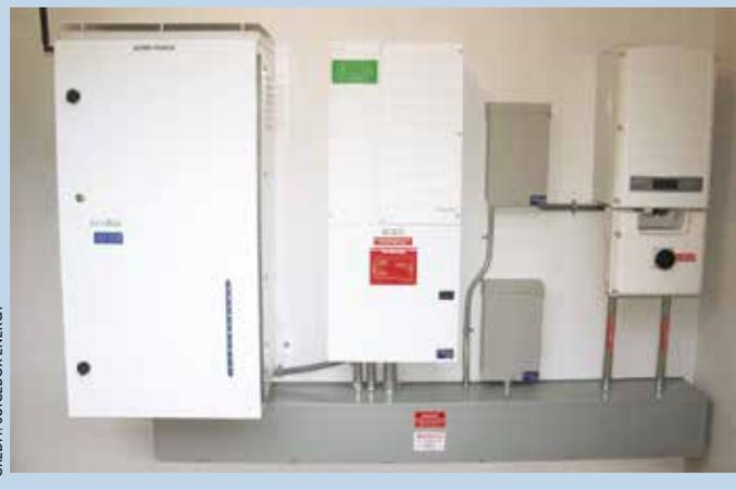
**JuiceBox Specs.** A 8.6-kWh lithium-ion battery pack with proprietary charge control and energy management system is coupled to the Schneider Conext *XW+* inverter, which is now listed and approved for use in Hawaii.
